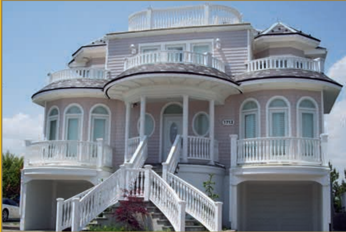
Above photo shows the use of Spectis custom radius rails and twisted radius stair rails along with top & bottom rails and newel posts with caps
